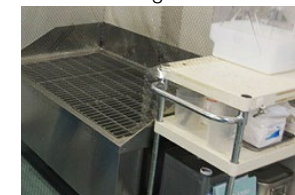
Washstand for waste liquid equipped with purification processing equipment
